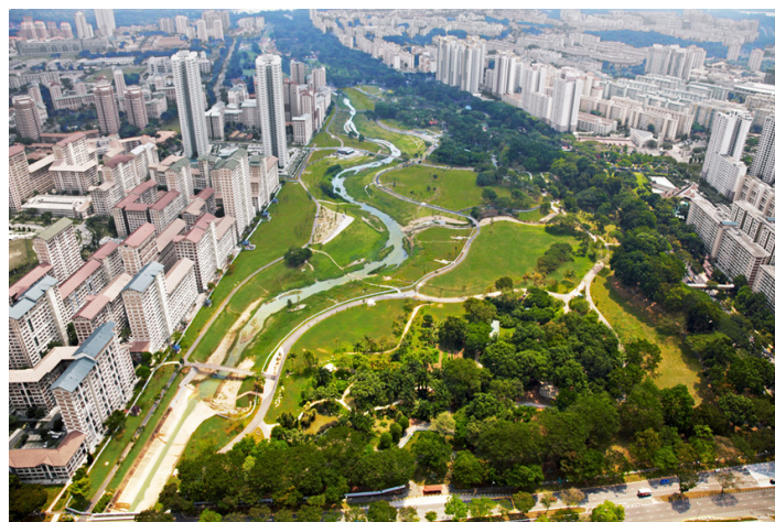
Figure 1. Bishan-Ang Mo Kio Park (Singapore) was delivered by a partnership between the Parks Department and the Water Agency. Source: Pagodashophouse on Wikimedia Commons [CC BY-SA 3.0 ( https://creativecommons.org )]
