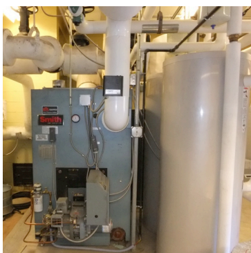
Figure 7. Heating Oil Backup System
