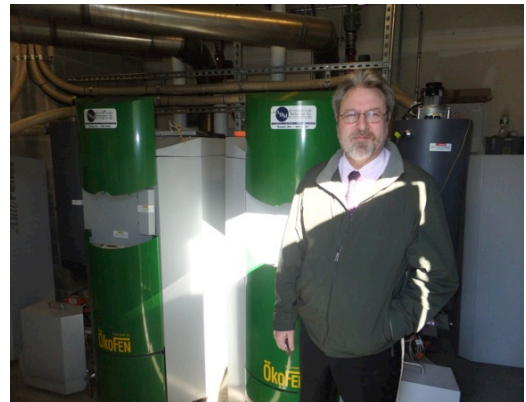
Figure 3. Kenneth Coville by ÖkoFEN Pellet Boilers
