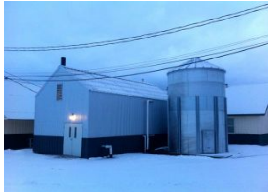
Figure 16. Pellet Silo and Boiler Housing Building. (photo by Wisewood Inc)
