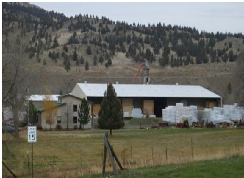
Figure 19. Malheur Lumber Yard
