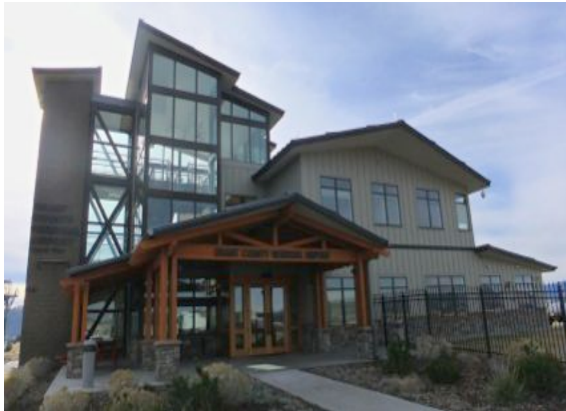
Figure 10. Grant County Regional Airport Airbase Building
